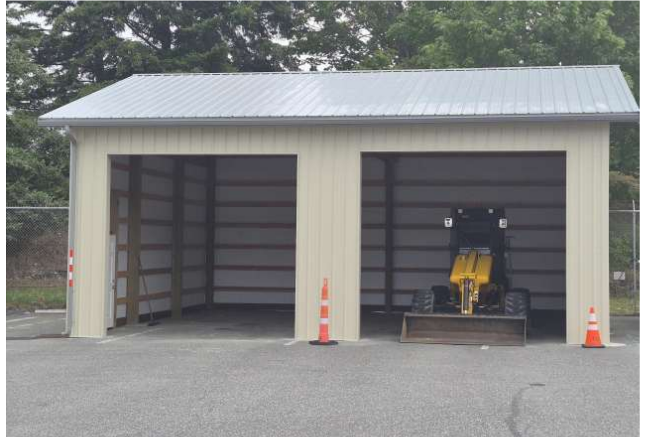
Ops covered storage near completion
