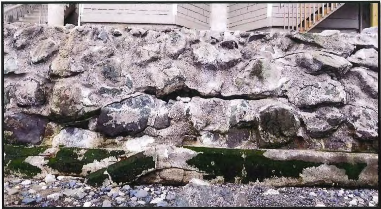
Dowell Existing Bulkhead (from shoreline) – Facing Northeast
