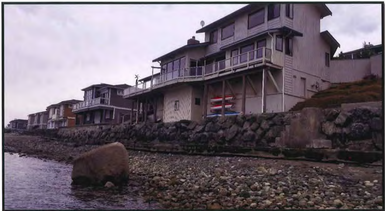
Foster Existing Bulkhead and Residence (from shoreline)
