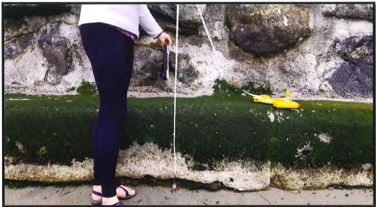
Dowell Existing Bulkhead (from shoreline) – Facing Northeast
