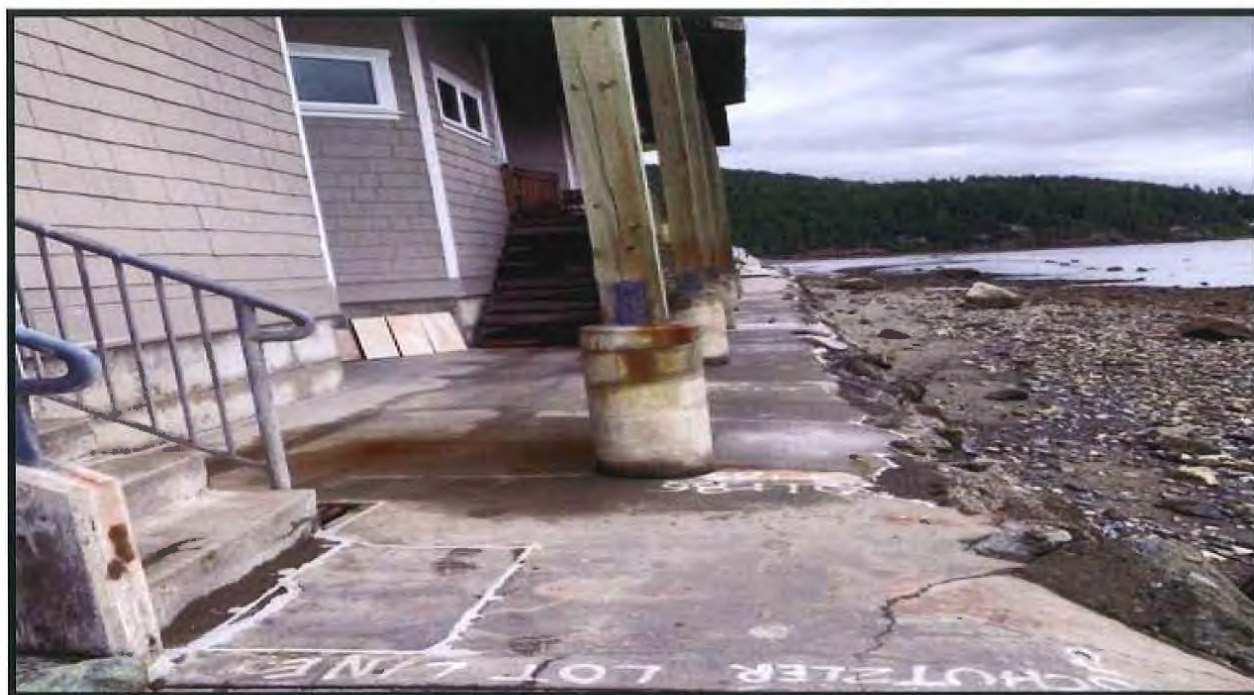
Schutzler Existing Bulkhead and Residence – Facing Southeast
