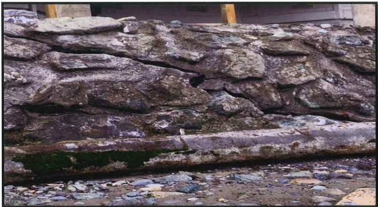
Schutzler Existing Bulkhead (from shoreline) – Facing East
