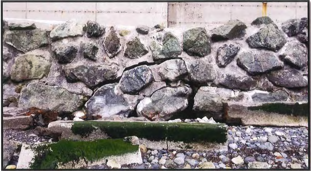
Dowell Existing Bulkhead (from shoreline) – Facing Northeast
