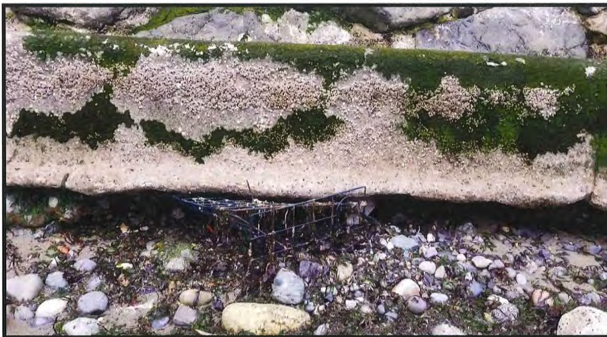
Foster Undercut Existing Bulkhead (from shoreline) – Facing Northeast
