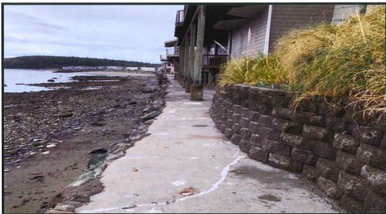
Schutzler Existing Bulkhead and Residence – Facing Northwest
