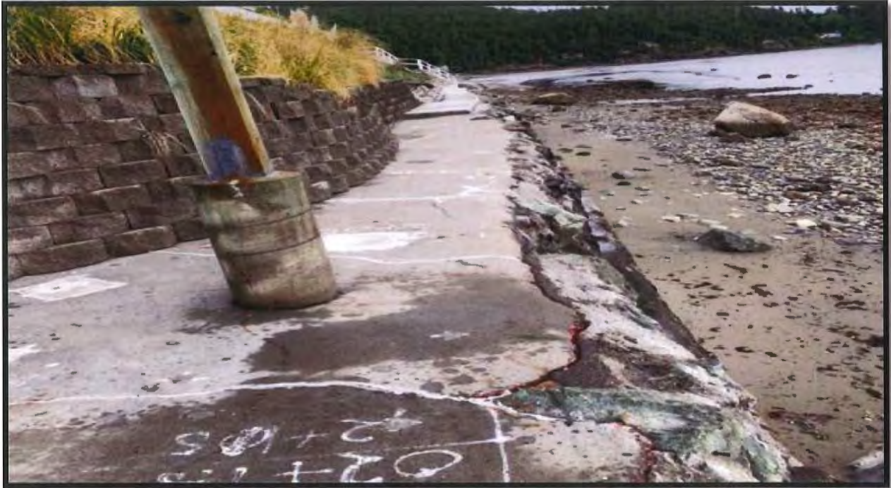
Schutzler Existing Bulkhead– Facing Southeast
