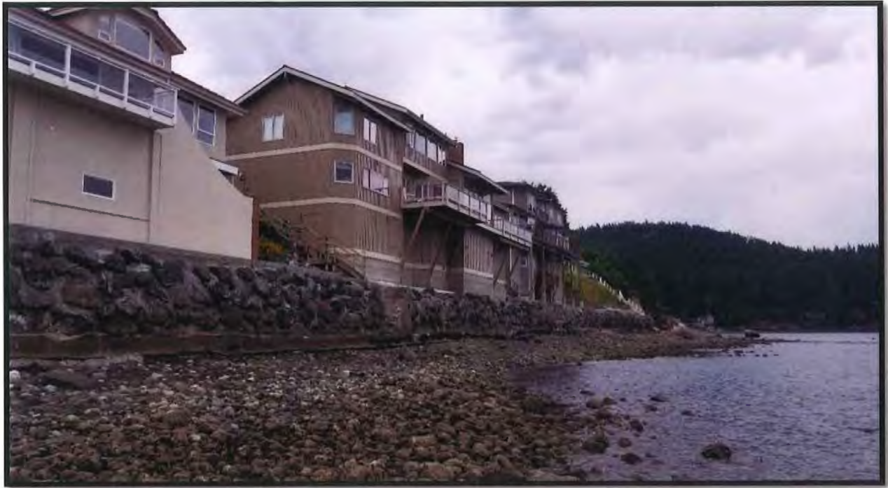
Dowell and Schutzler Residences – Facing Southeast
