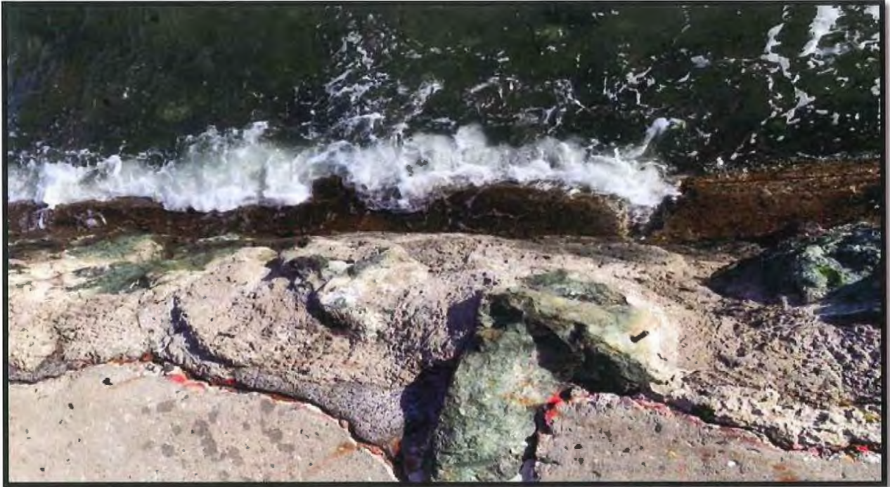
Dowell Existing Bulkhead (during high-tide)
