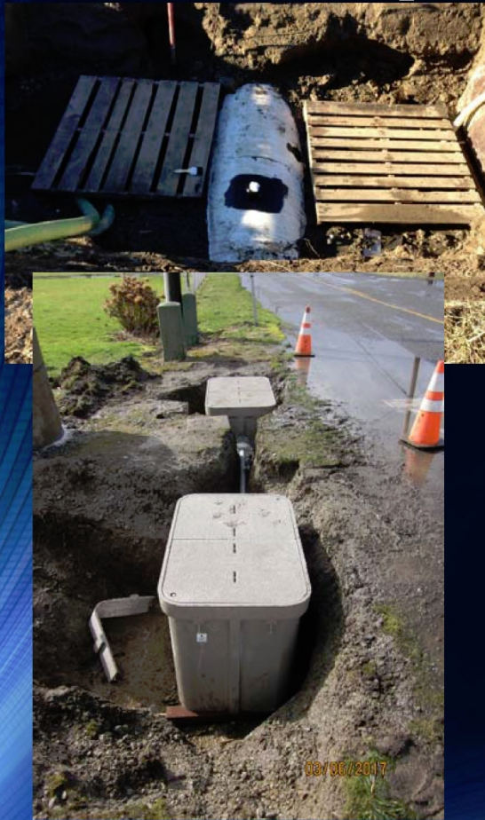
The crew installing breakouts for pipe in pipe
