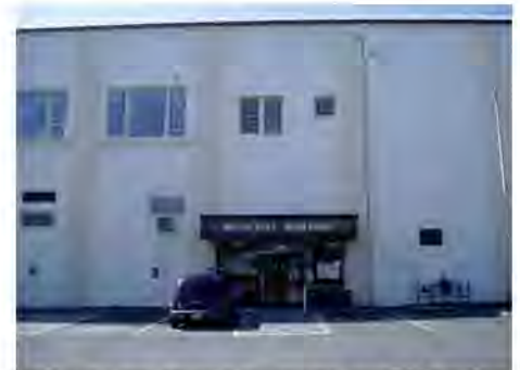
Parking Lot Entrance (North Side)
