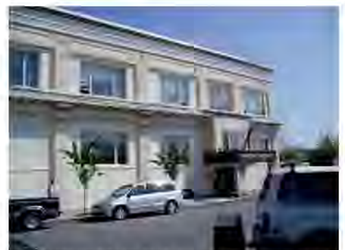
Existing Main Entrance (South side)
