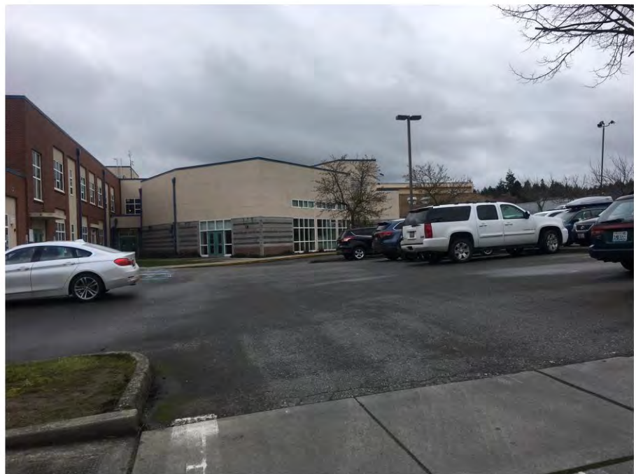
Existing AMS & ASD parking lot located off of 22 nd Street.
