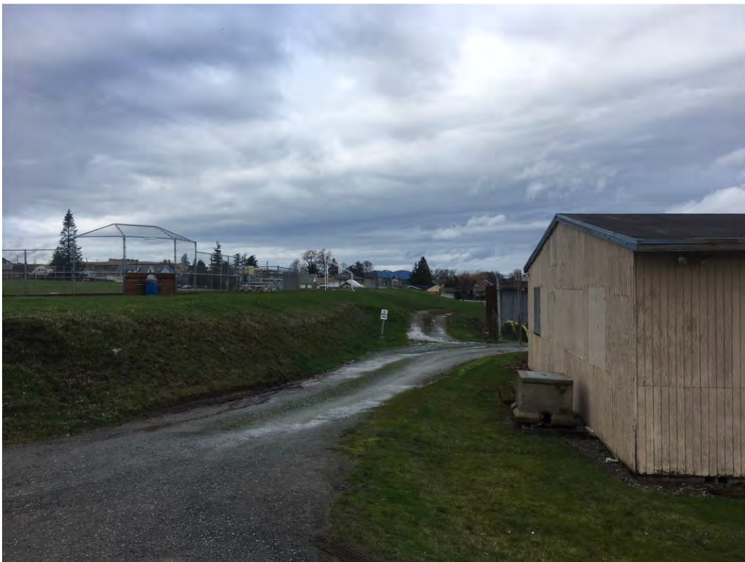
West side of maintenance building. Looking north approximately.
