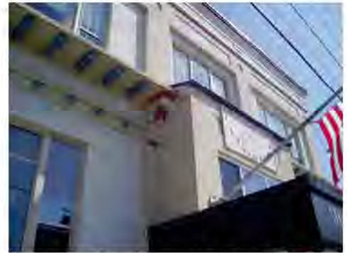
Entrance Front Façade (South Side)
