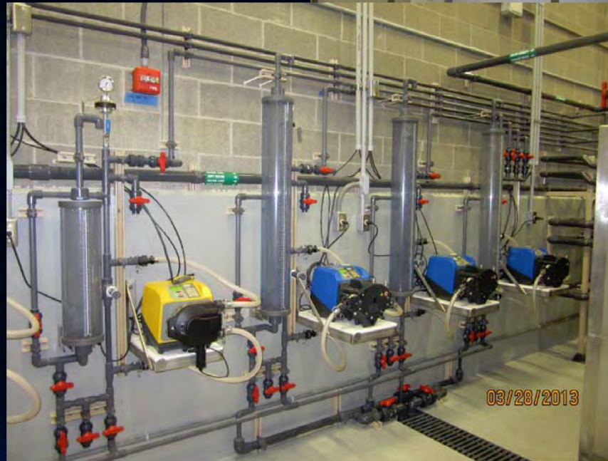
City of Anacortes water treatment plant existing chemical feed systems.
