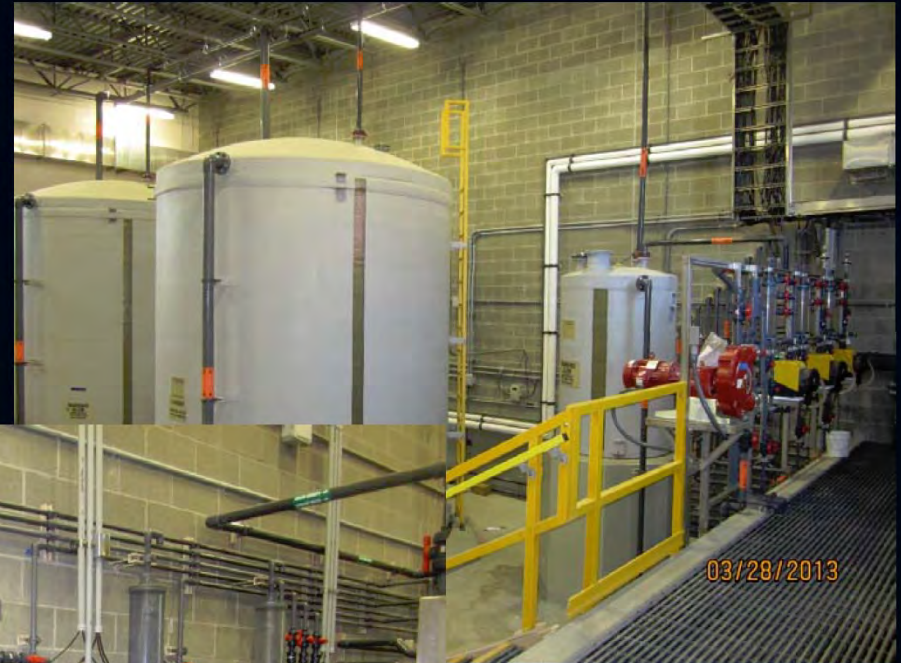
City of Anacortes water treatment plant existing chemical feed systems.
