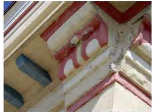
Exterior Plaster Column Capital
