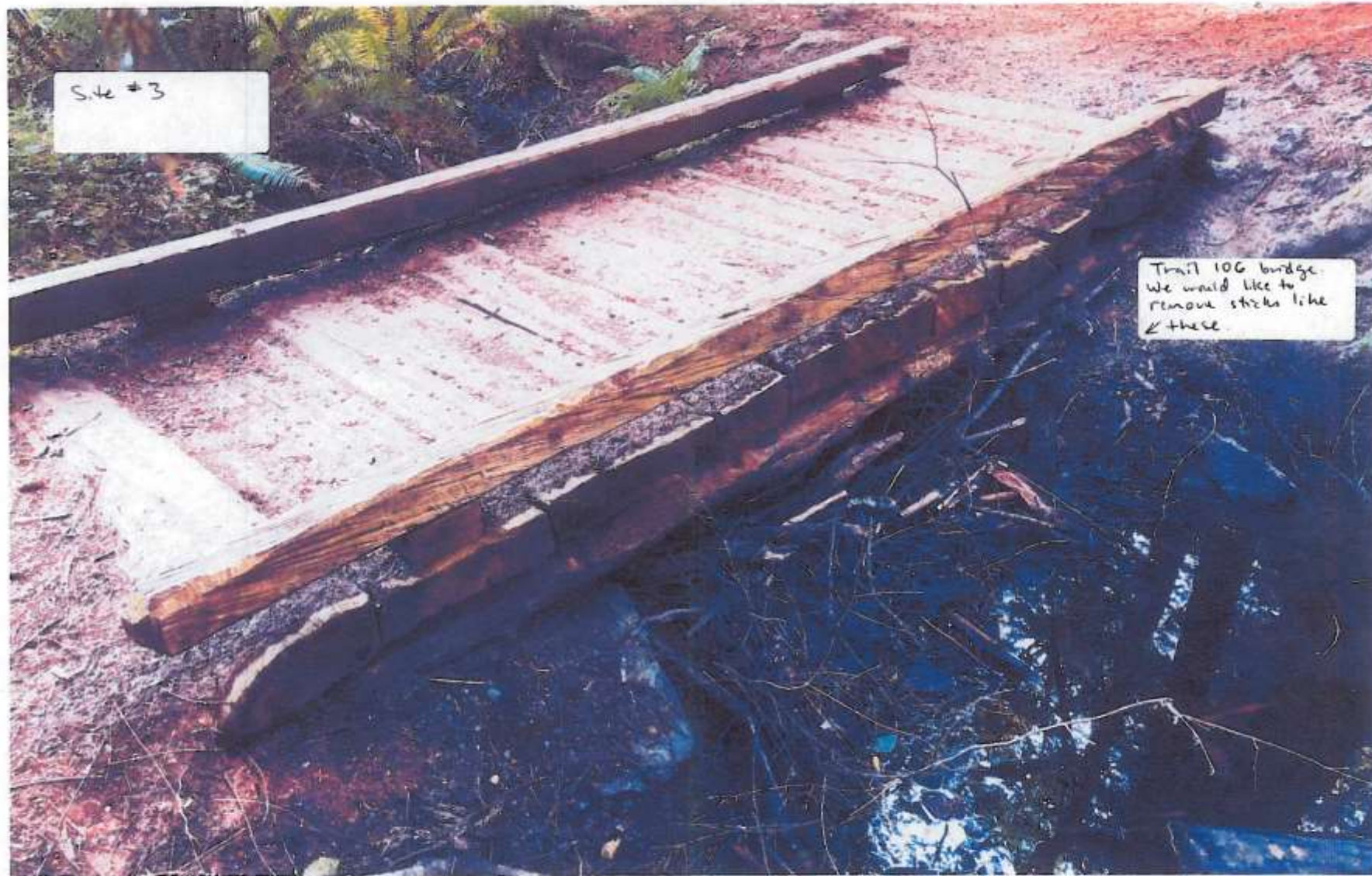
Site 3: Trail 106. Logs and sticks put under ACFL bridges by the beavers.
