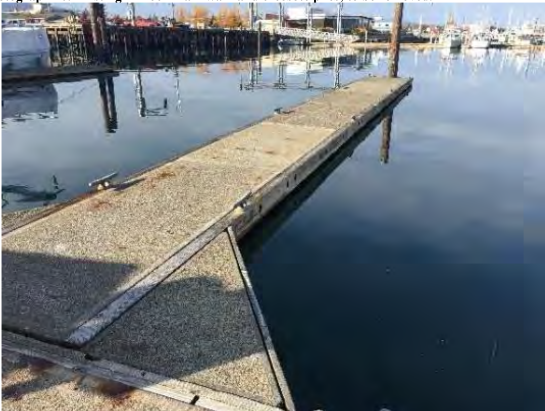
Photograph 11. Existing A-Dock finger, finger triangles, and creosote piles; to be removed.
