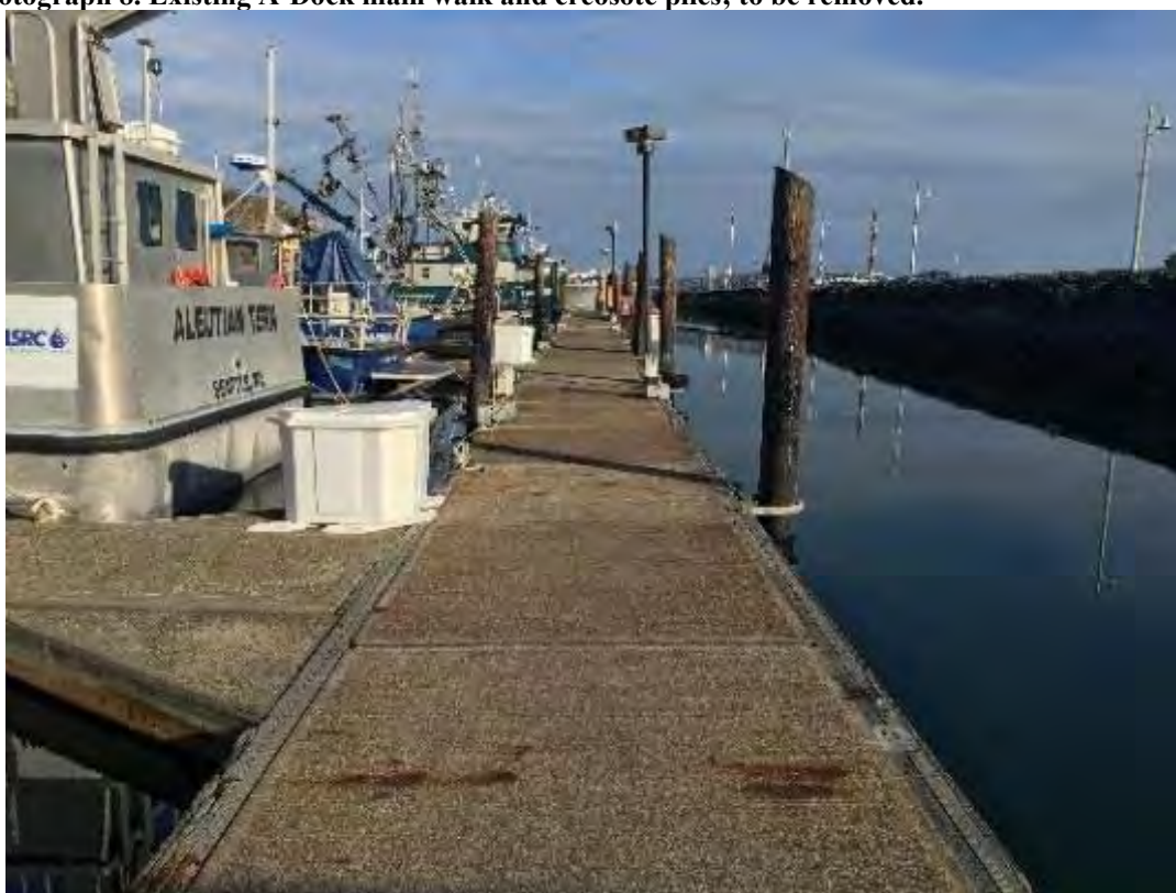
Photograph 9. Existing A-Dock main walk and creosote piles; to be removed.
