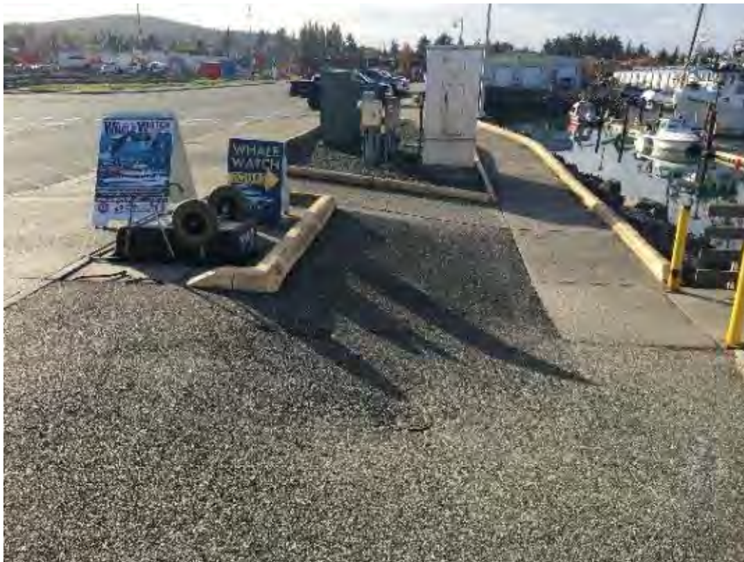
Photograph 1. Existing upland access to A-Dock that will be demolished and reconstructed for dock entrance.
