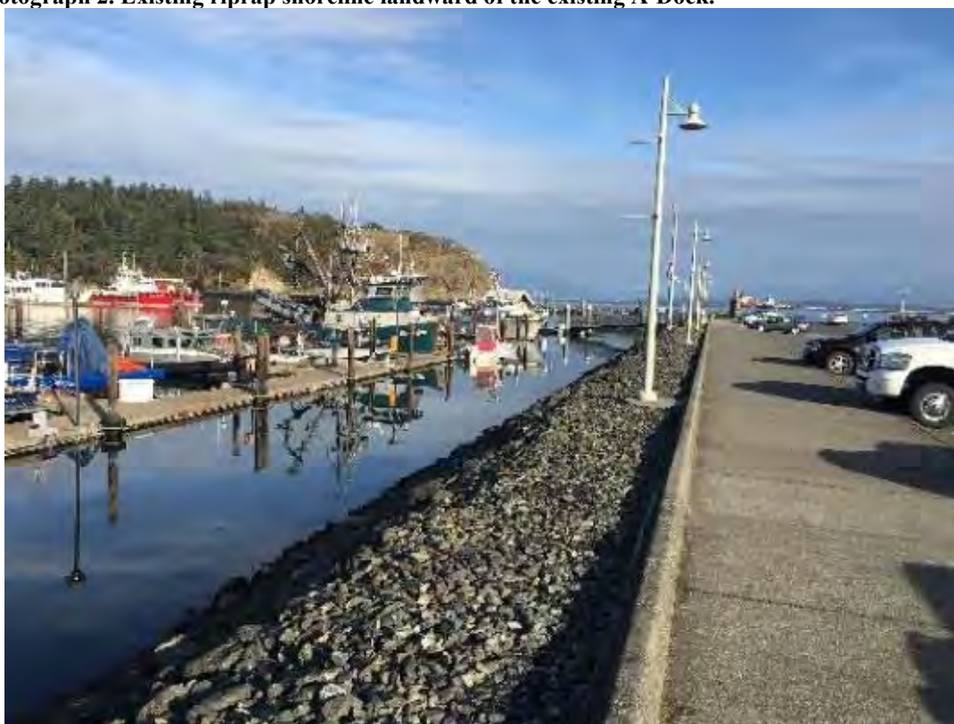
Photograph 3. Existing riprap shoreline landward of the existing A-Dock and concrete sidewalk.
