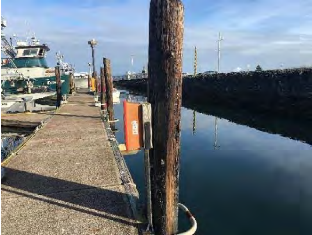
Photograph 10. Existing A-Dock main walk and creosote piles; to be removed.
