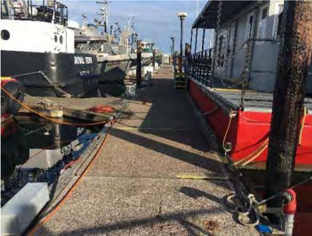
Photograph 6. Existing A-Dock main walk and creosote piles; to be removed.
