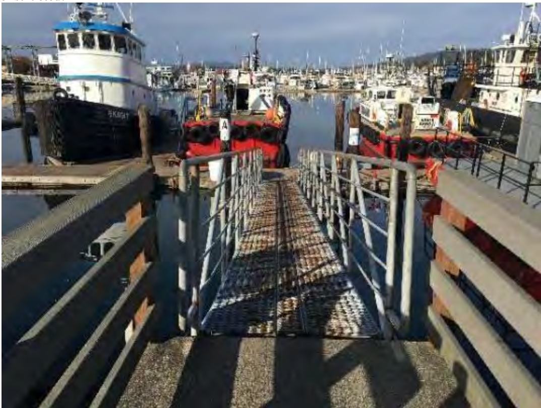
Photograph 5. Existing concrete abutment and gangway to A-Dock; to be removed and demolished.
