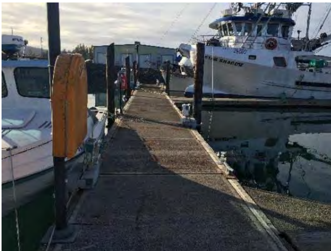
Photograph 8. Existing A-Dock main walk and creosote piles; to be removed.
