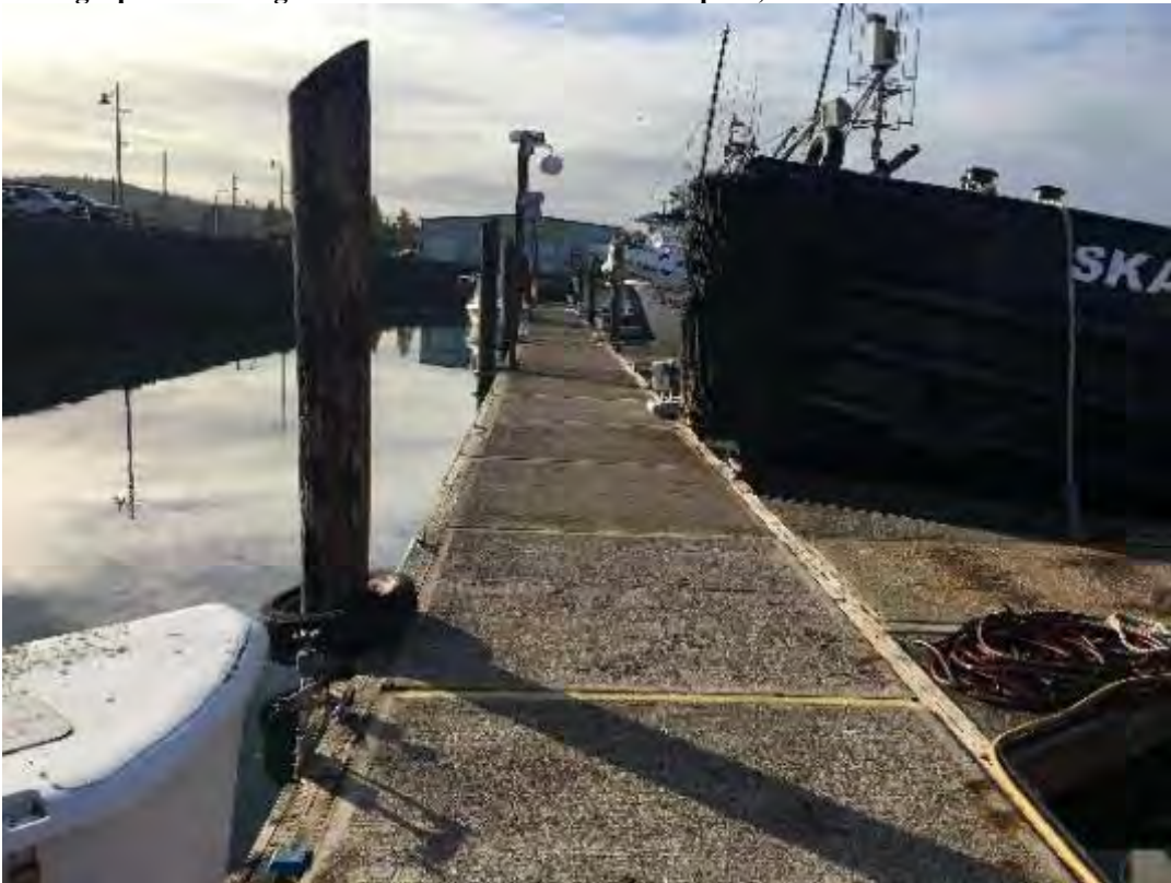
Photograph 7. Existing A-Dock main walk and creosote piles; to be removed.
