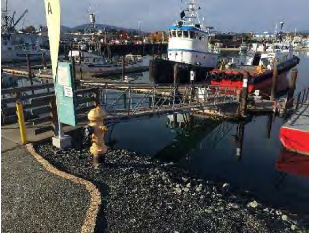
Photograph 4. Existing concrete abutment and gangway to A-Dock; to be demolished and reconstructed.
