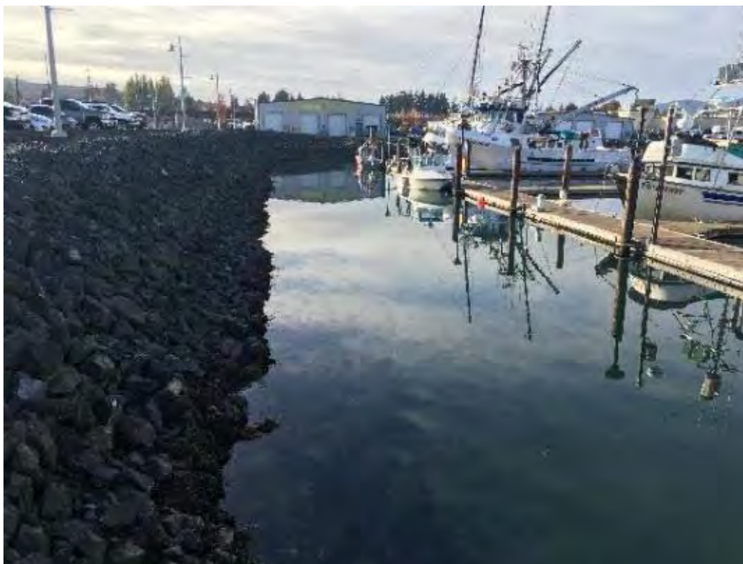
Photograph 2. Existing riprap shoreline landward of the existing A-Dock.
