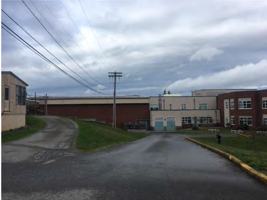
Looking north at AMS. East side of maintenance building is located on the left side. Proposed building would be behind maintenance building.
