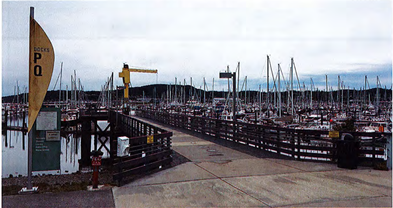
Photograph 1. South facing view of P/Q Pier and crane (06/12/18).
