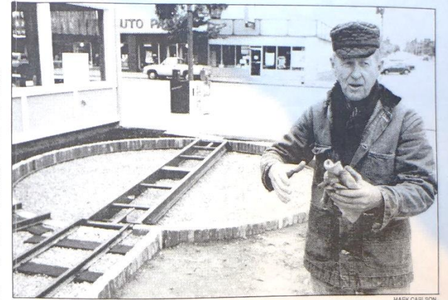
Tommy Thompson, alongside the locomotive turntable on Ninth Street, describes how the engine will glide around on ballbearings at the mere touch of a finger. He predicts completion of the project by the Fourth of July.
