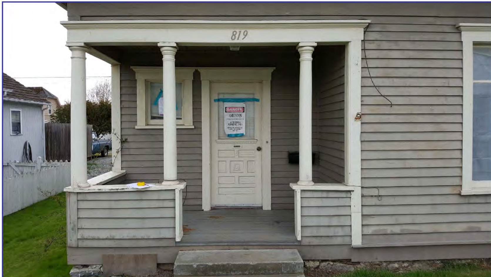
“At Home in Anacortes” 1904 house demolished March 2017
