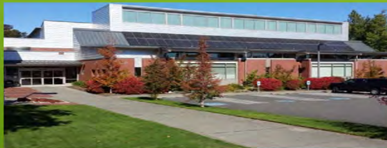
Library 17.28 solar array
