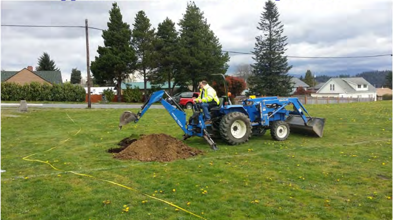
Photo A: Location of TP-1 and site surface conditions. Photo looking north by northeast.
