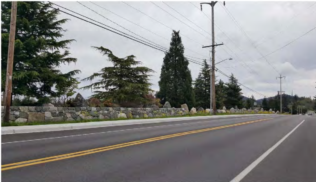
D Ave. looking south (4/19/17)
