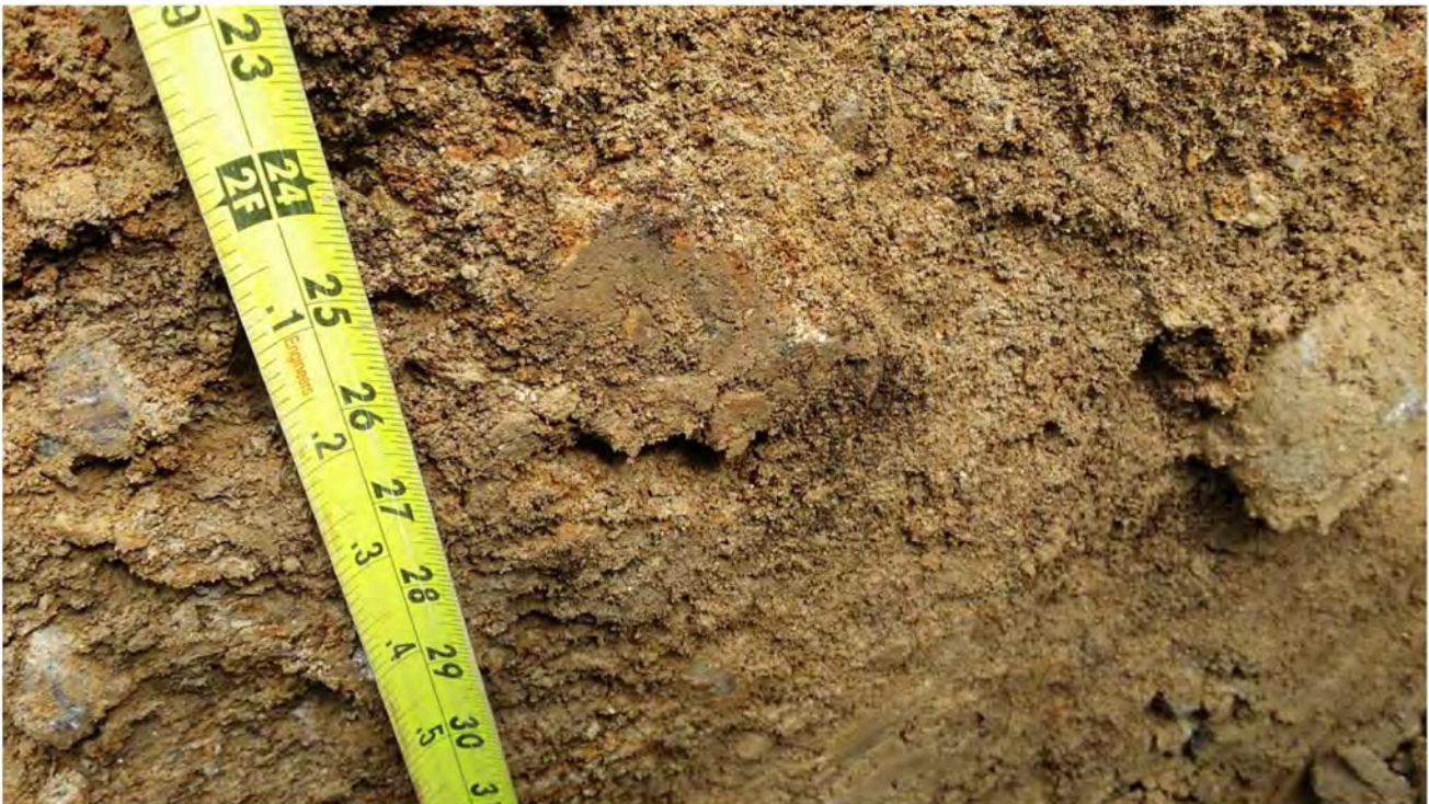
Photo B: Detail of weathered native glacial drift soils at TP-1 at about 2.0 feet BPG. Note rust colored mottling, moisture content and fine-grained texture..
