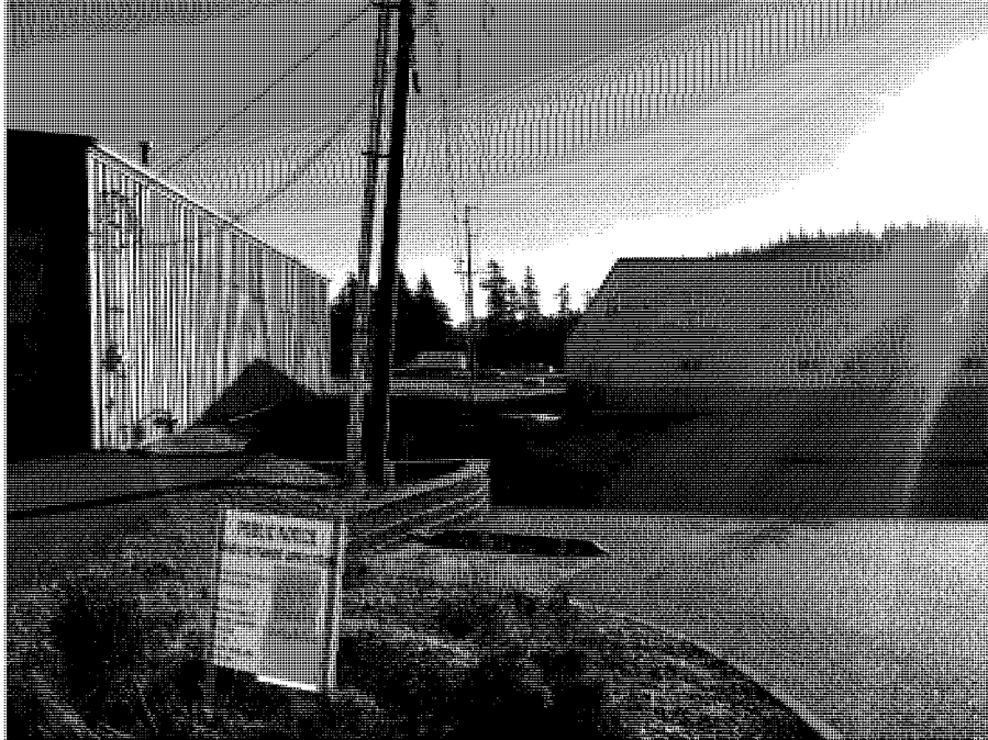
East side of subject building located in background. Looking south toward SR20. Neighboring commercial business located on left side of picture.
