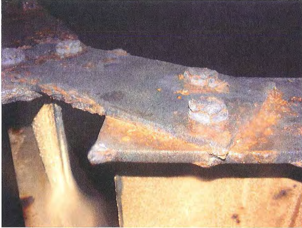
FIGURE 3 Connection at Top of W16 Girders
