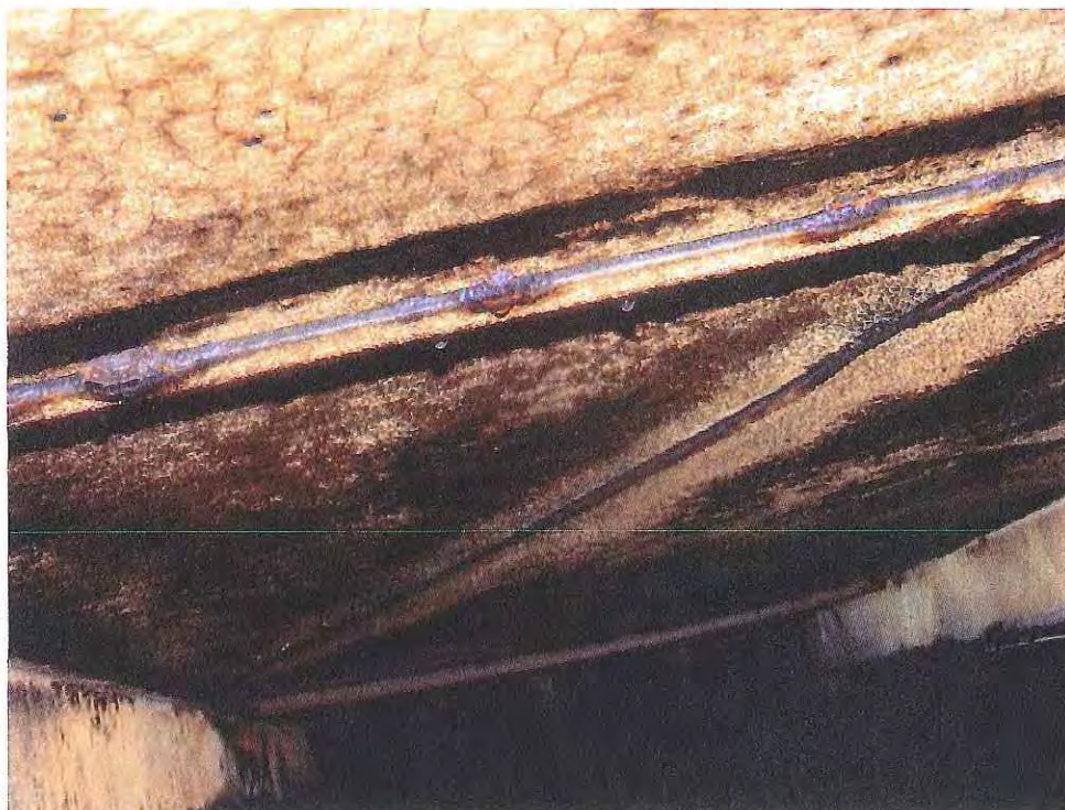
FIGURE 28 Steel Bar Running Between W8 Beams
