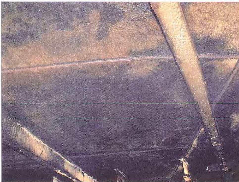
FIGURE 32 Typical Roof Plate Condition Near Center of Reservoir
