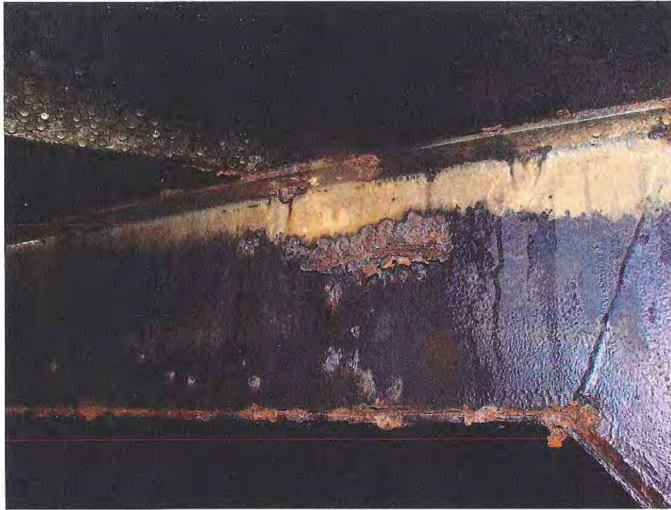
FIGURE 19 W10 Beam Near Perimeter of Tank
