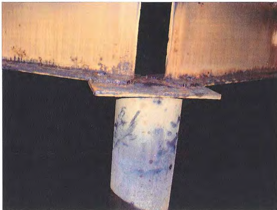
FIGURE 2 Top of an Intermediate Column and Bearing Point of W16 Girders
