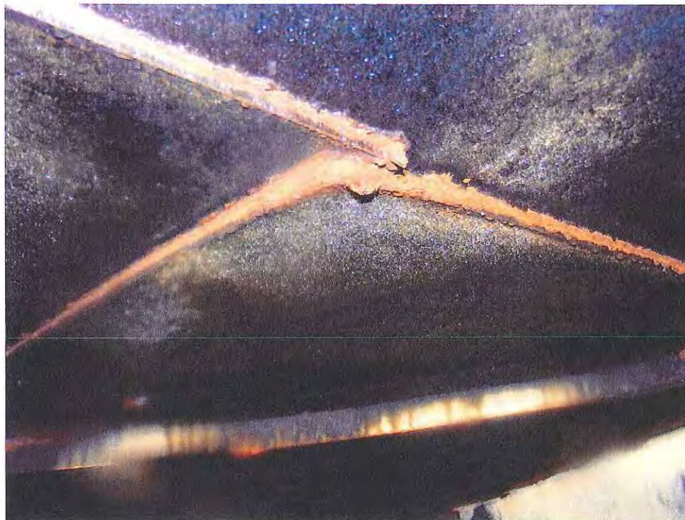
FIGURE 34 Typical Roof Plate Condition Near Perimeter of Reservoir
