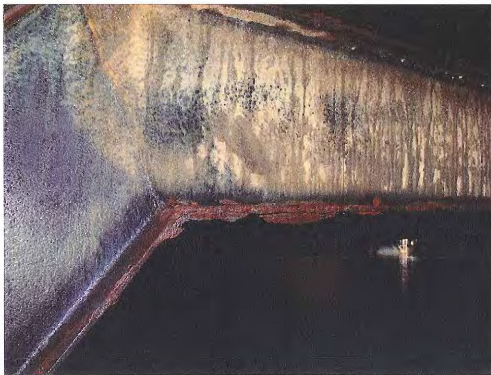
FIGURE 18 W10 Beam Near Perimeter of Tank
