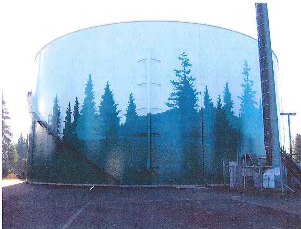
FIGURE 37 Reservoir with Spiral Access Stairway
