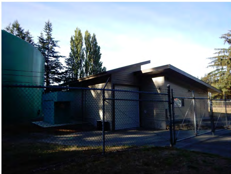
Photo 4. Booster pump station within the project site, looking southwest from Blue Heron Circle
