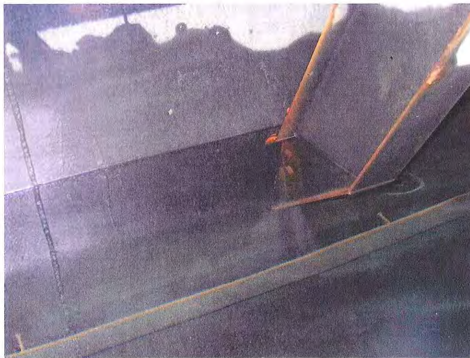
FIGURE 20 W10 Connection to Tank Shell
