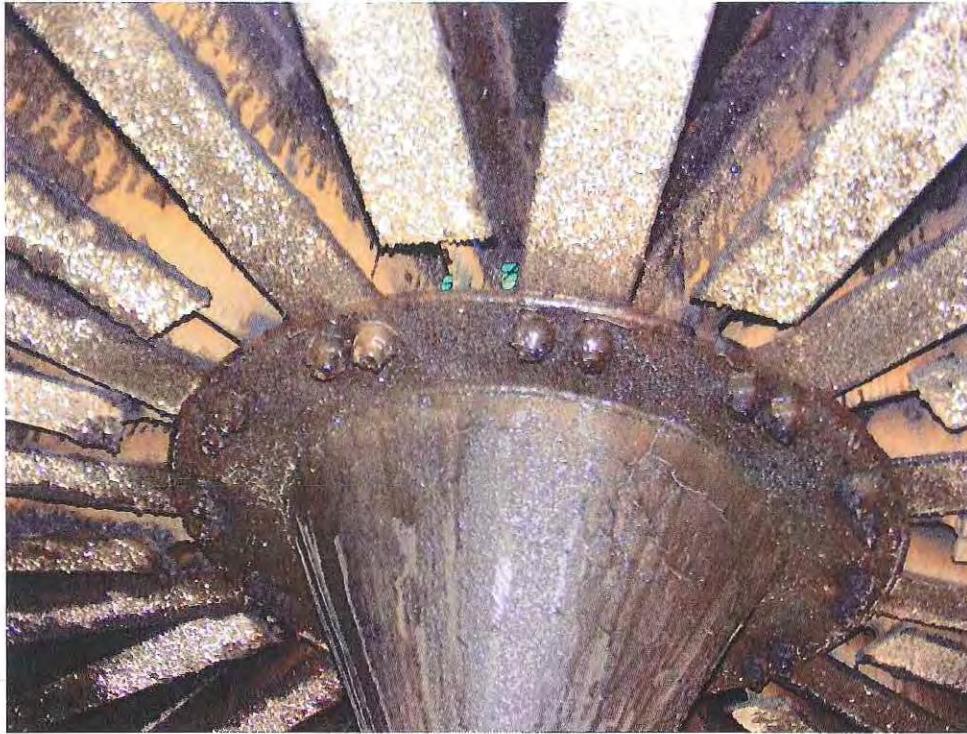
FIGURE 1 Top of Center Column
