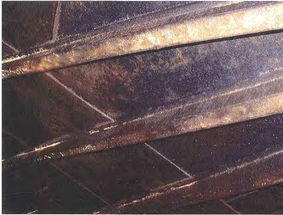
FIGURE 31 Typical Roof Plate Condition Near Center of Reservoir
