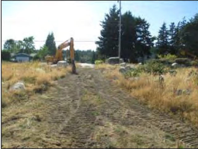
#1 – Looking east over the south portion of the site near the 31 st Street right of way to be vacated.
