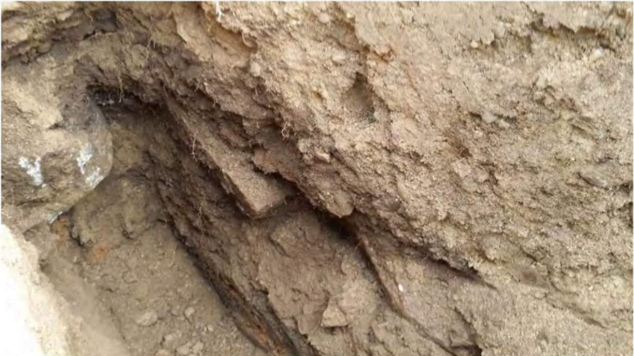
Photo F: Excavation of TP-3 at termination depth showing highly variable uncontrolled fills persisting to end depth.
