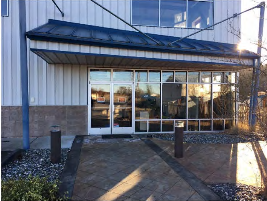
Front building entrance.
