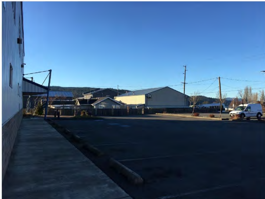
Looking west at front of subject commercial building.
