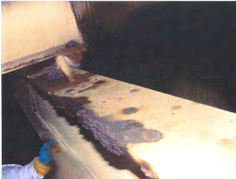
FIGURE 5 Top of a W16 Girder Near a W8 Connection
