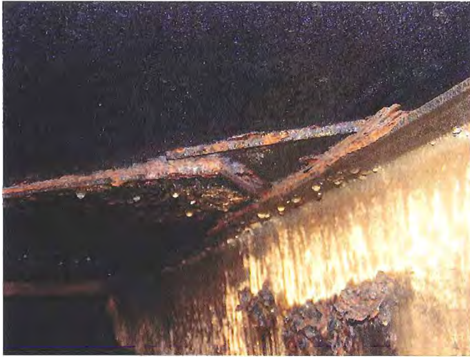
FIGURE 35 Typical Roof Plate Condition Near Perimeter of Reservoir
