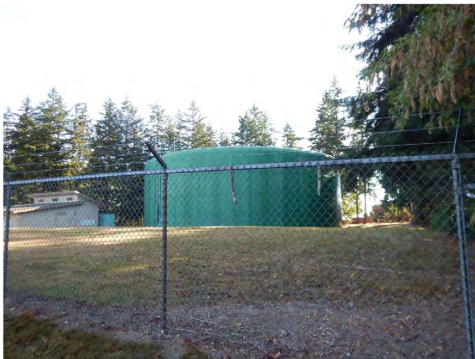
Photo 1. View of the existing water reservoir and new water reservoir site, looking east from Whistle Lake Road
