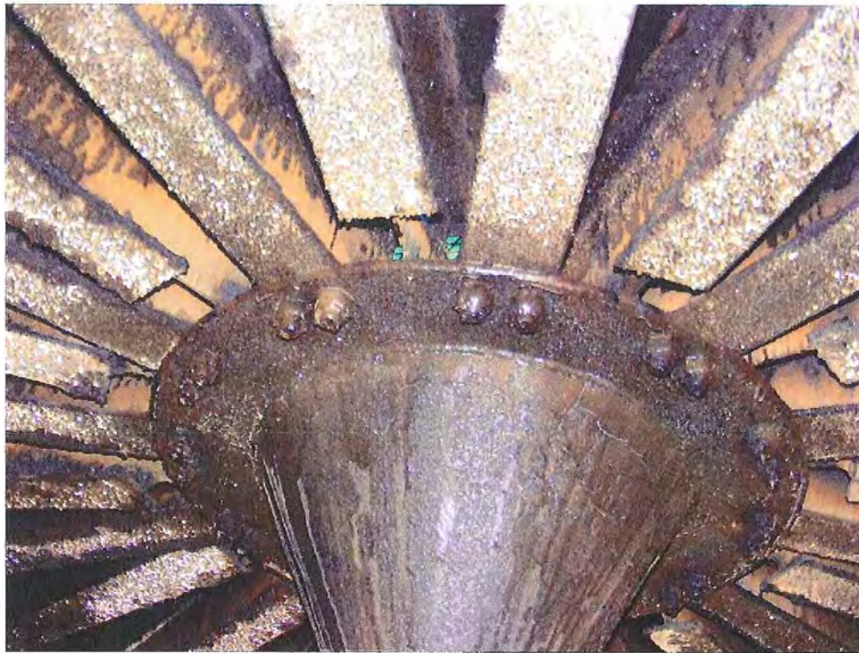
FIGURE 1 Top of Center Column
