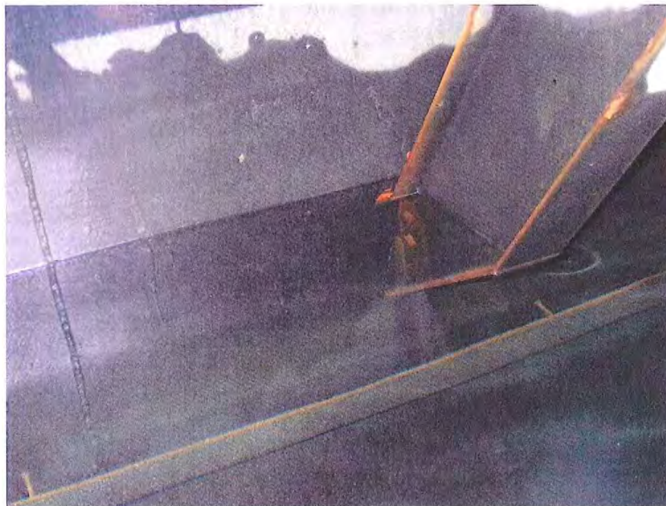
FIGURE 20 W10 Connection to Tank Shell
