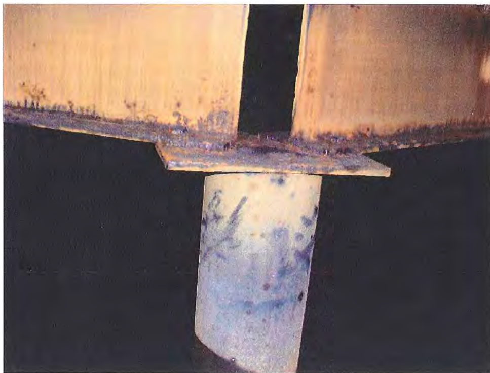
FIGURE 2 Top of an Intermediate Column and Bearing Point of W16 Girders
