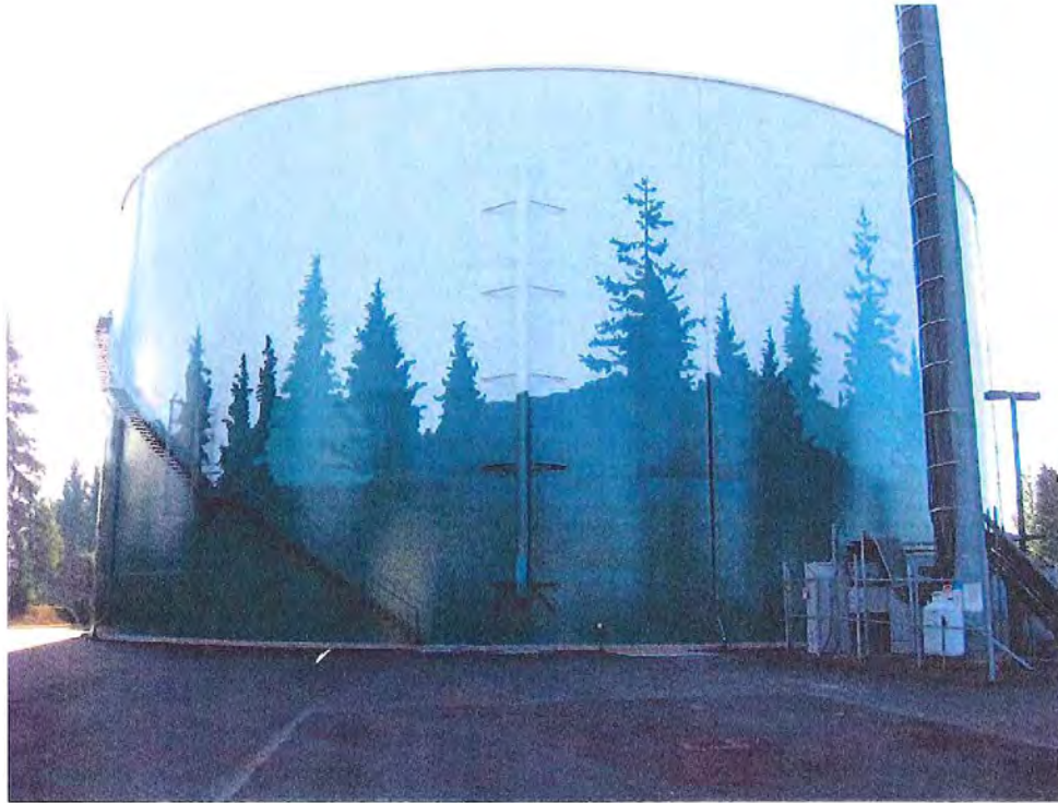
FIGURE 37 Reservoir with Spiral Access Stairway
