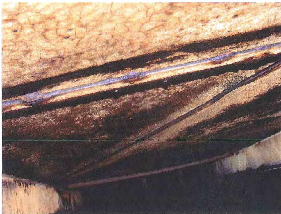
FIGURE 28 Steel Bar Running Between W8 Beams
