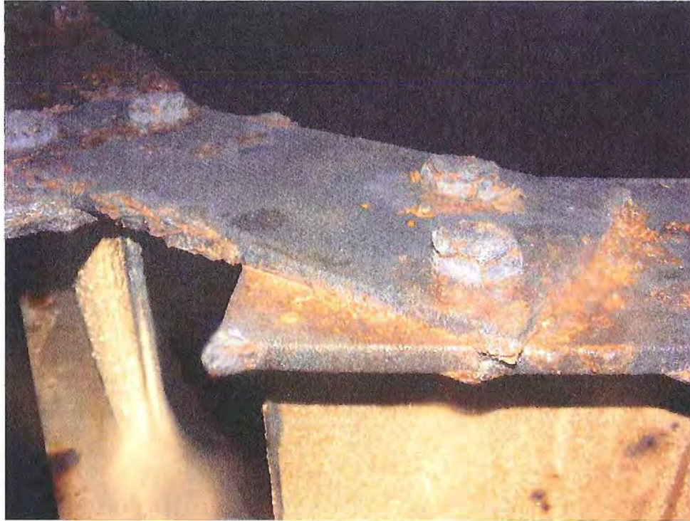
FIGURE 3 Connection at Top of W16 Girders
