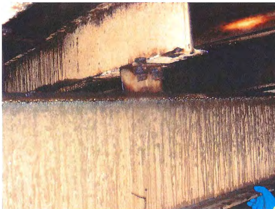
FIGURE 12 W8 Connection to W16
