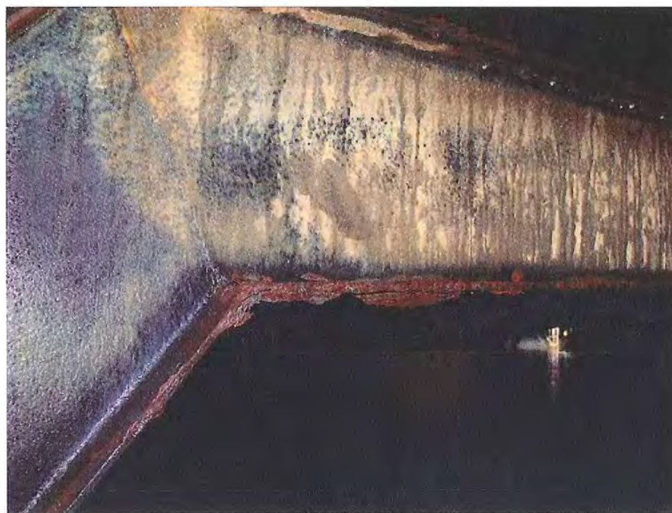
FIGURE 18 W10 Beam Near Perimeter of Tank
