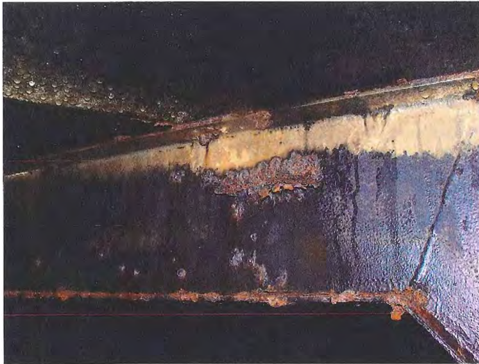
FIGURE 19 W10 Beam Near Perimeter of Tank
