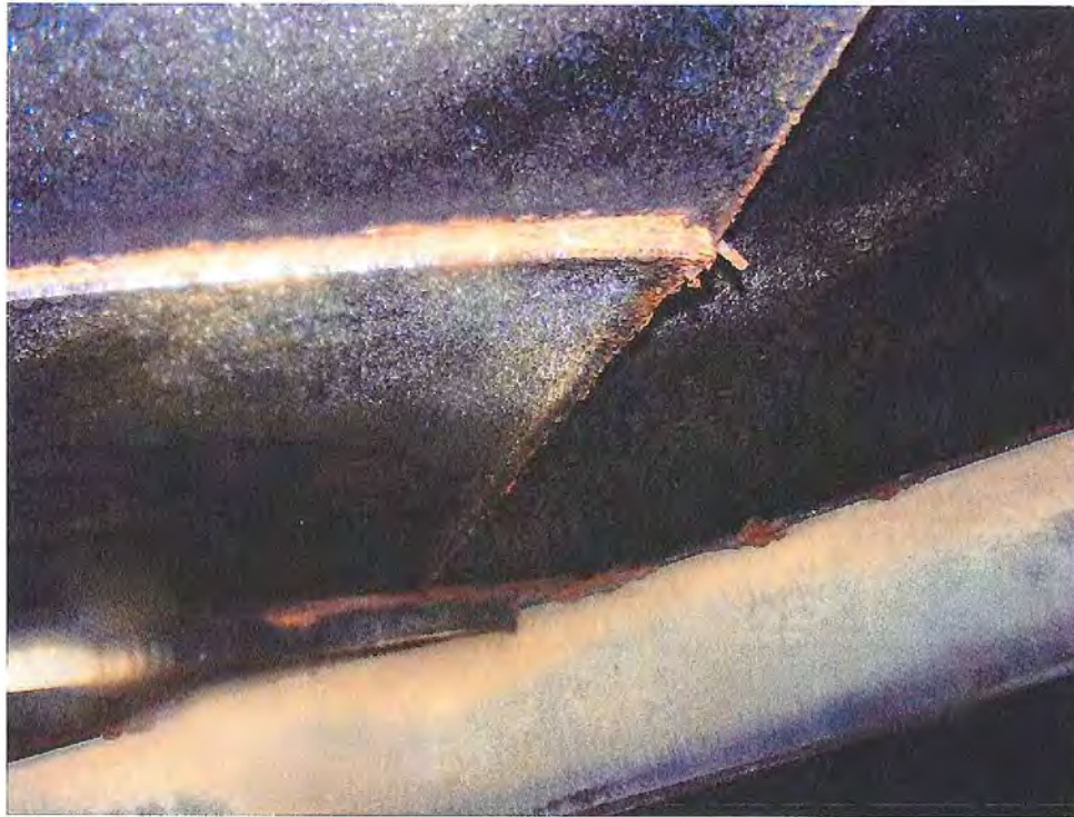
FIGURE 33 Typical Roof Plate Condition Near Perimeter of Reservoir
