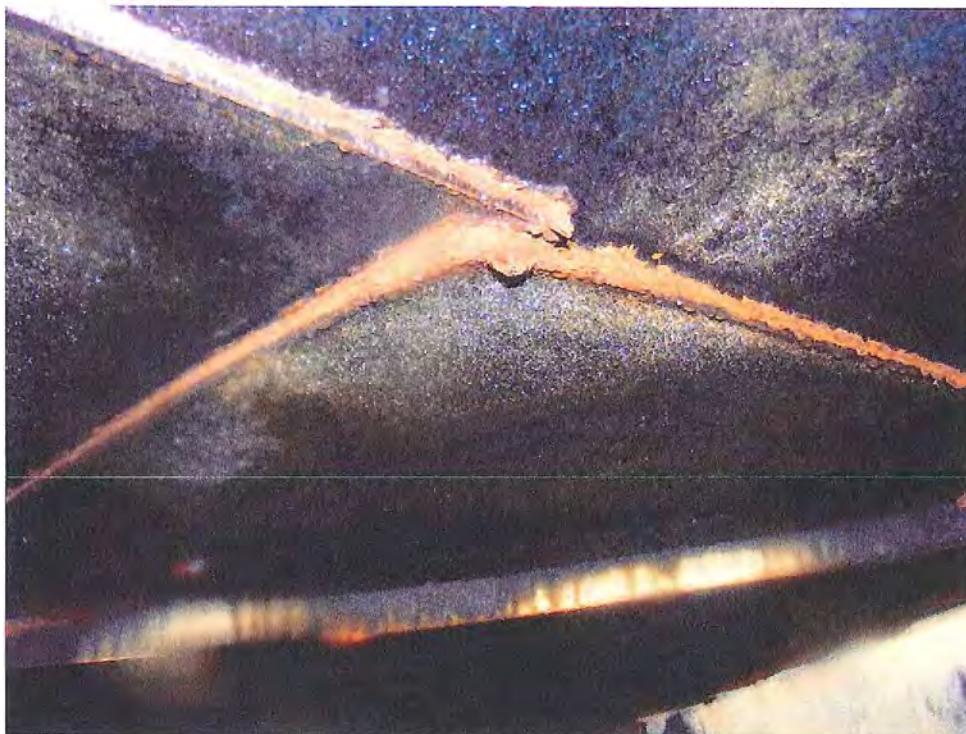
FIGURE 34 Typical Roof Plate Condition Near Perimeter of Reservoir
