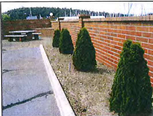
Photo 5. Existing non-native cypress shrubs provide limited habitat. Three native Pacific dogwood trees are proposed for installation in this area (Photo: AES, 5/11/2015).
