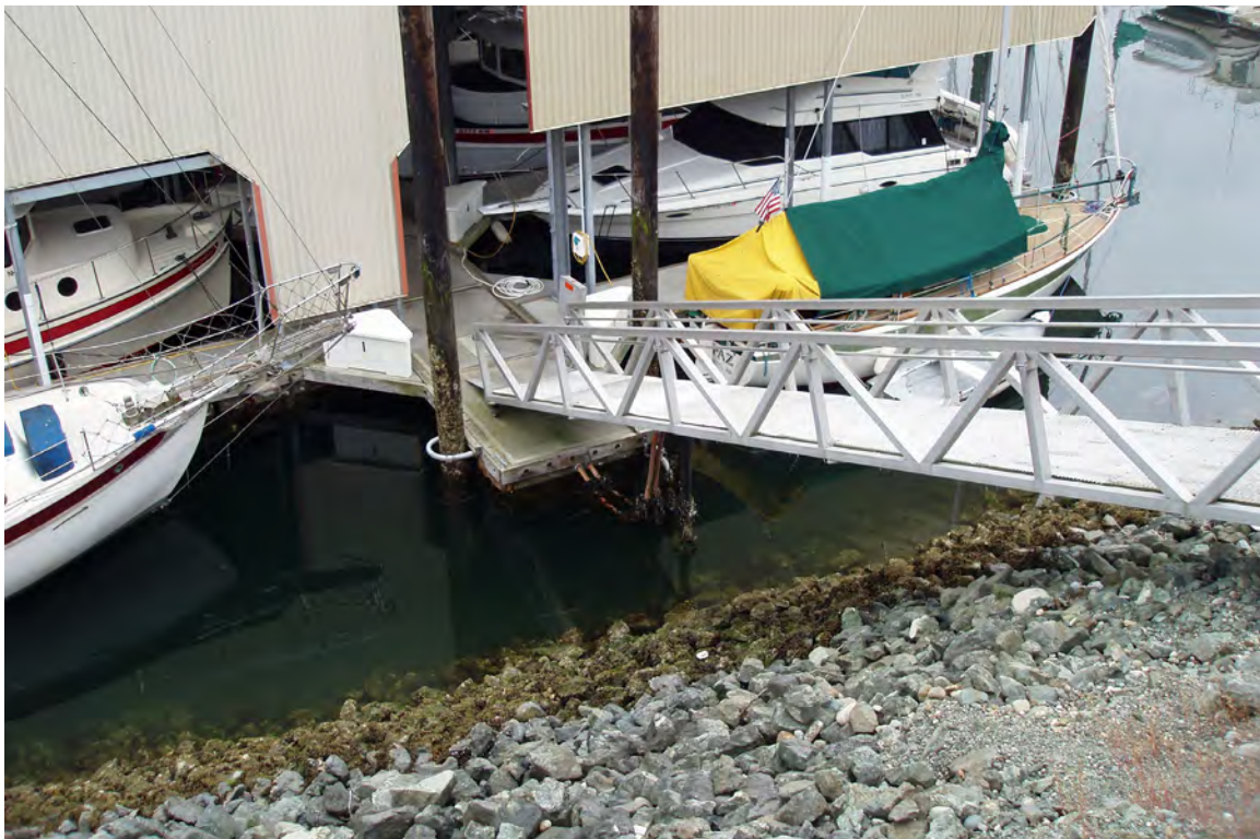
Figure 4. Anacortes Marina, top and bottom, rock riprap and existing gangways. A band of macroalgae, primarily Fucus and Ulva , is visible on the lower intertidal portion of the riprap. Notice the steep angles of the gangways. Photos 6/6/09, predicted tide -1.3 ft.
