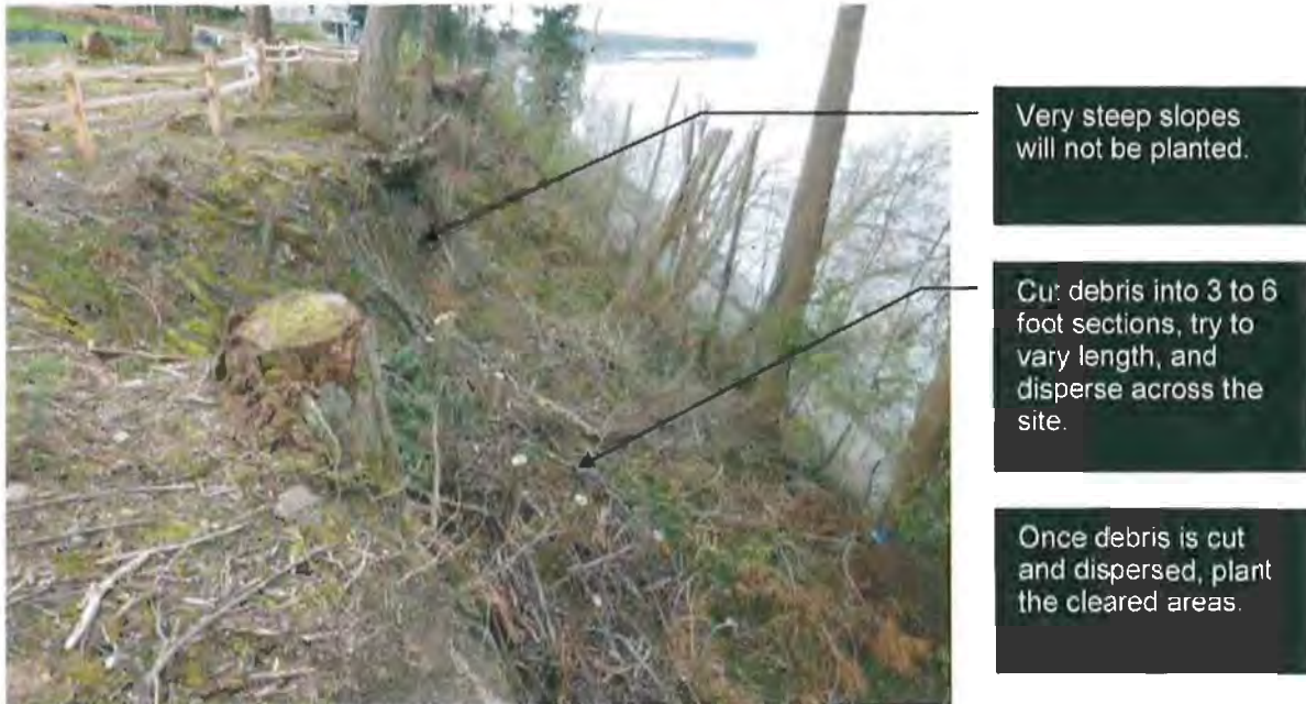
Photo 1: This is an example of 1.) Exposed soils (labelled) requiring erosion protection and planting; and 2.) Dense debris layers requiring cutting and dispersal across site, with follow-up planting required.
