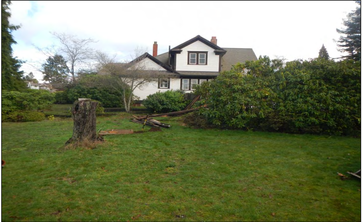
Photo 1. Overview, rear and south, of the residence from the orchard area.
