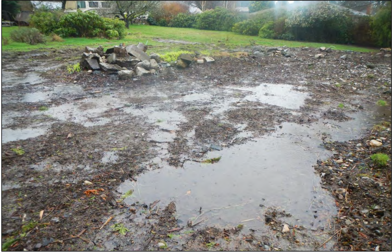
Photo 3. Demolished barn location; view west.
