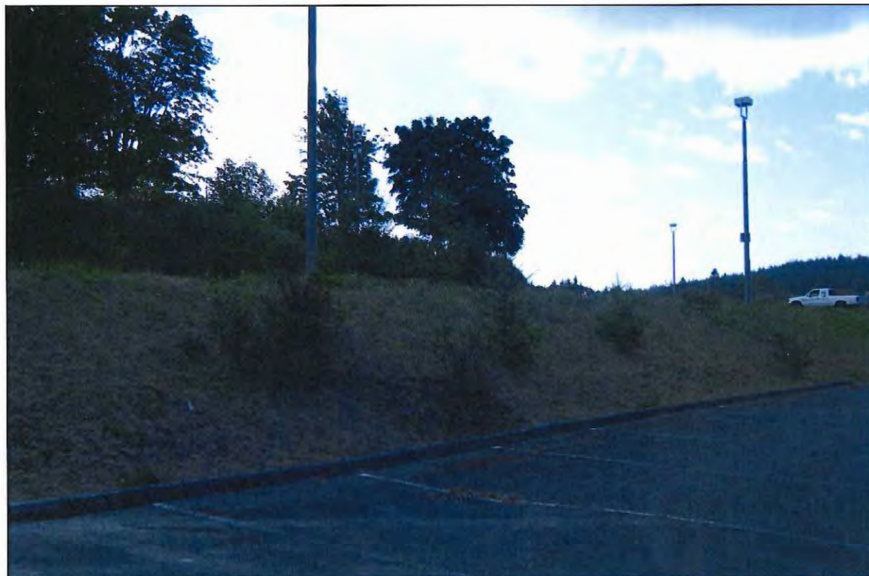
Photo 2. Example backfilled sediments in north parking lot
